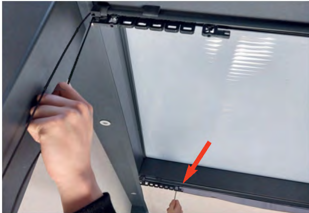
5.) Tension the system and readjust if required.
