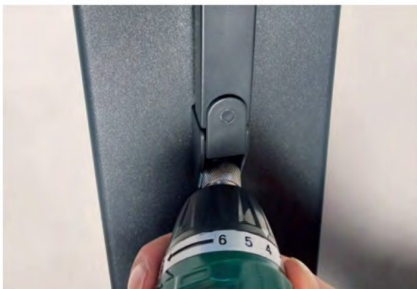
7.) Screw the spring tensioner tight accordingly.
