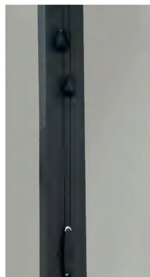
View of operating cord with operating handle and spring tensioner
